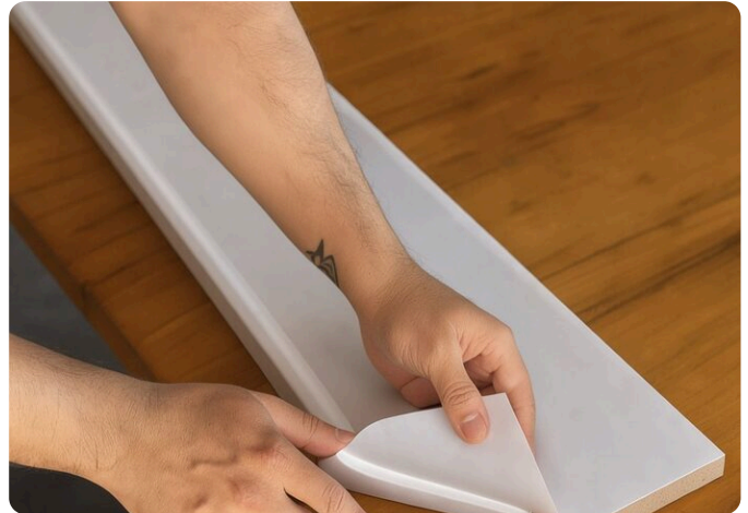
Peeling the liner off the adhesive film, on the back of the molding. Illustrative image.
